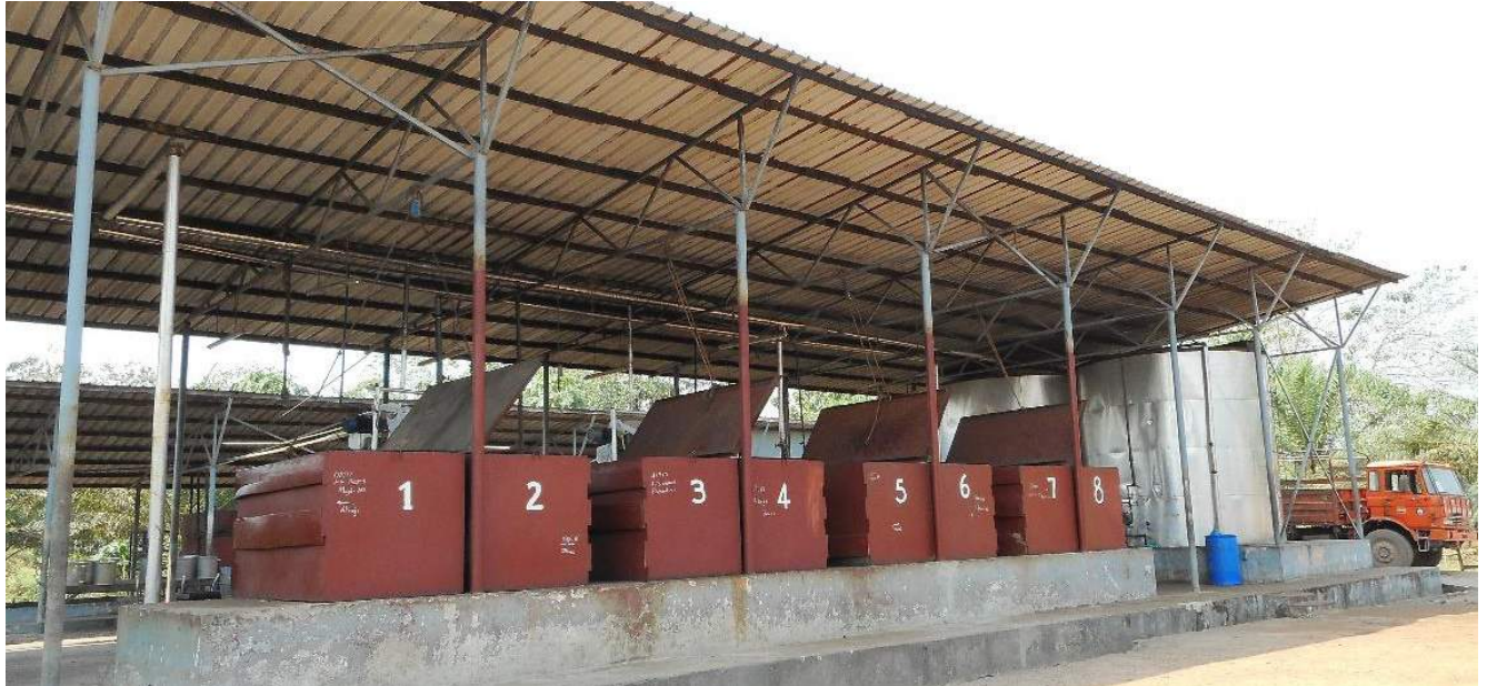
Figure 7 Nedoil CPO Mill
